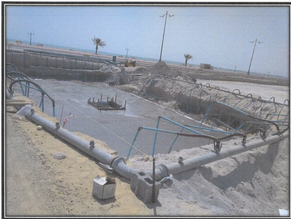
DEWATERING WORKS AT SHUBAILY @ QATIF
