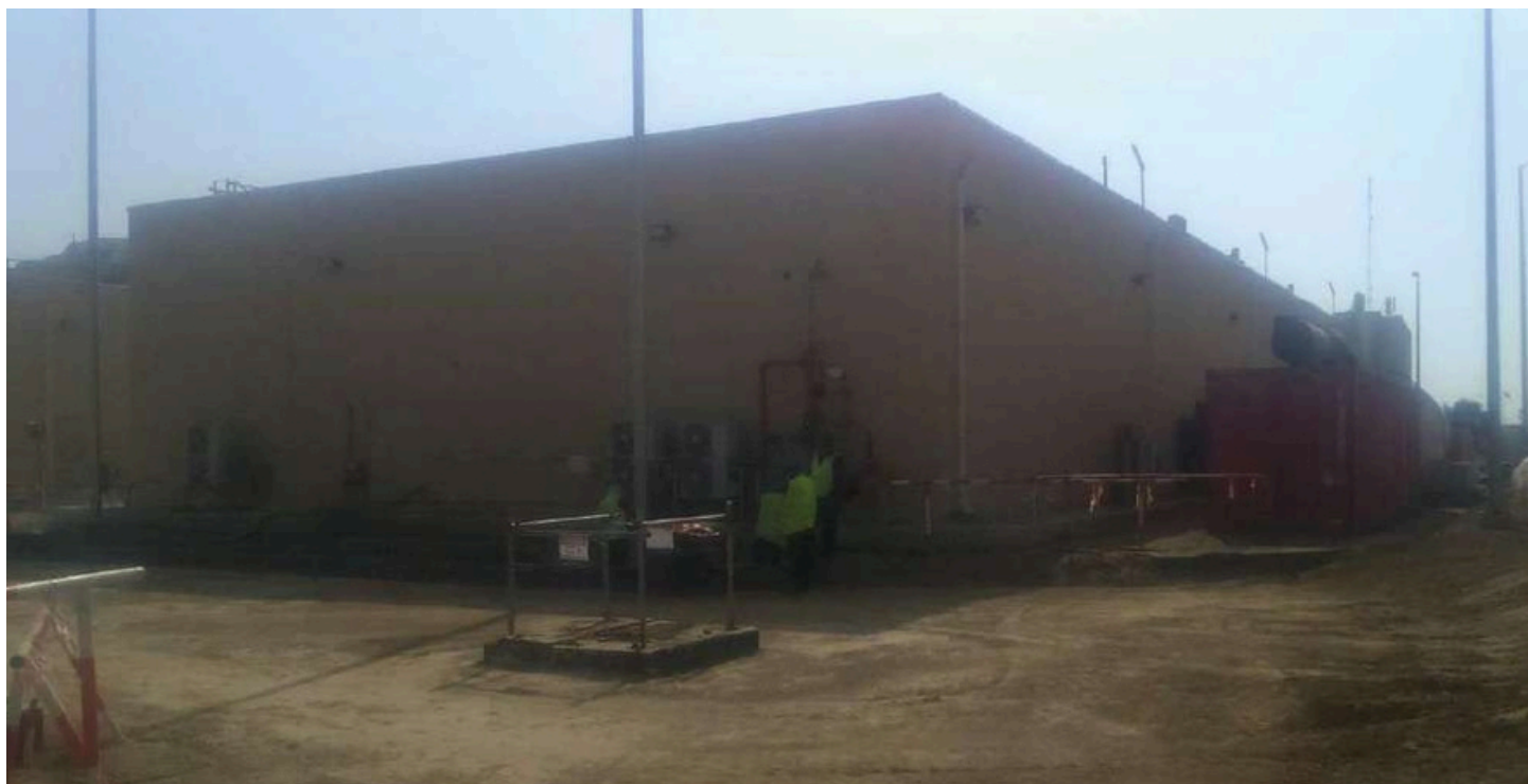
Control Building Site Preparation, Jazan IGCC
