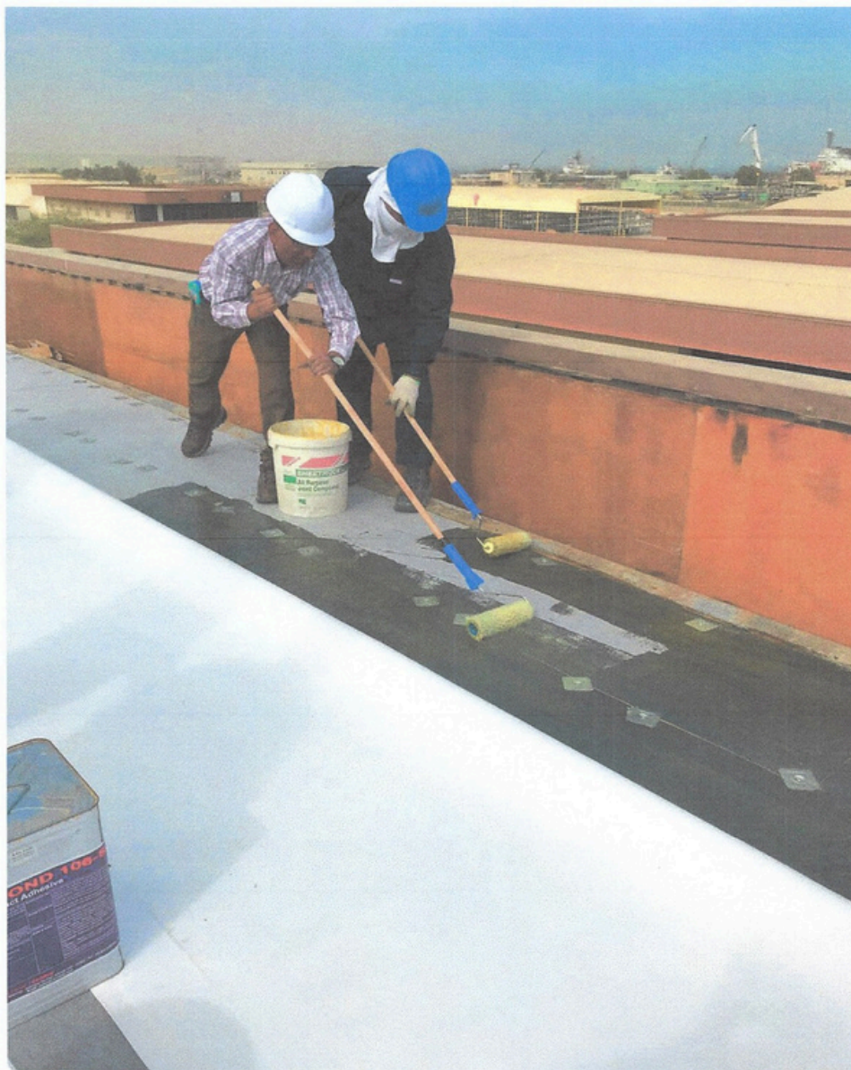
WATERPROOFING WORKS @ TANAJIB
