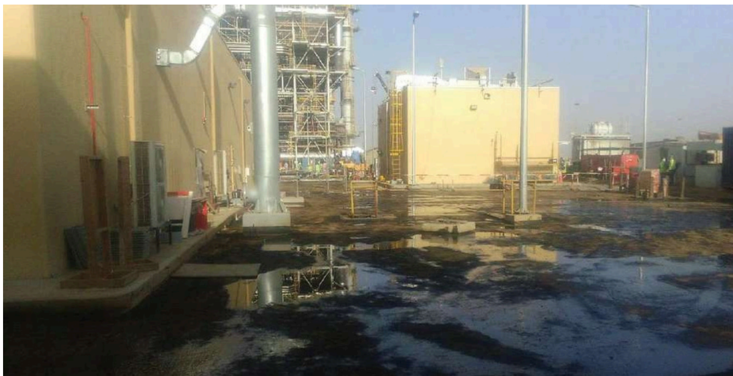
Control Building Road Paving, Jazan IGCC
