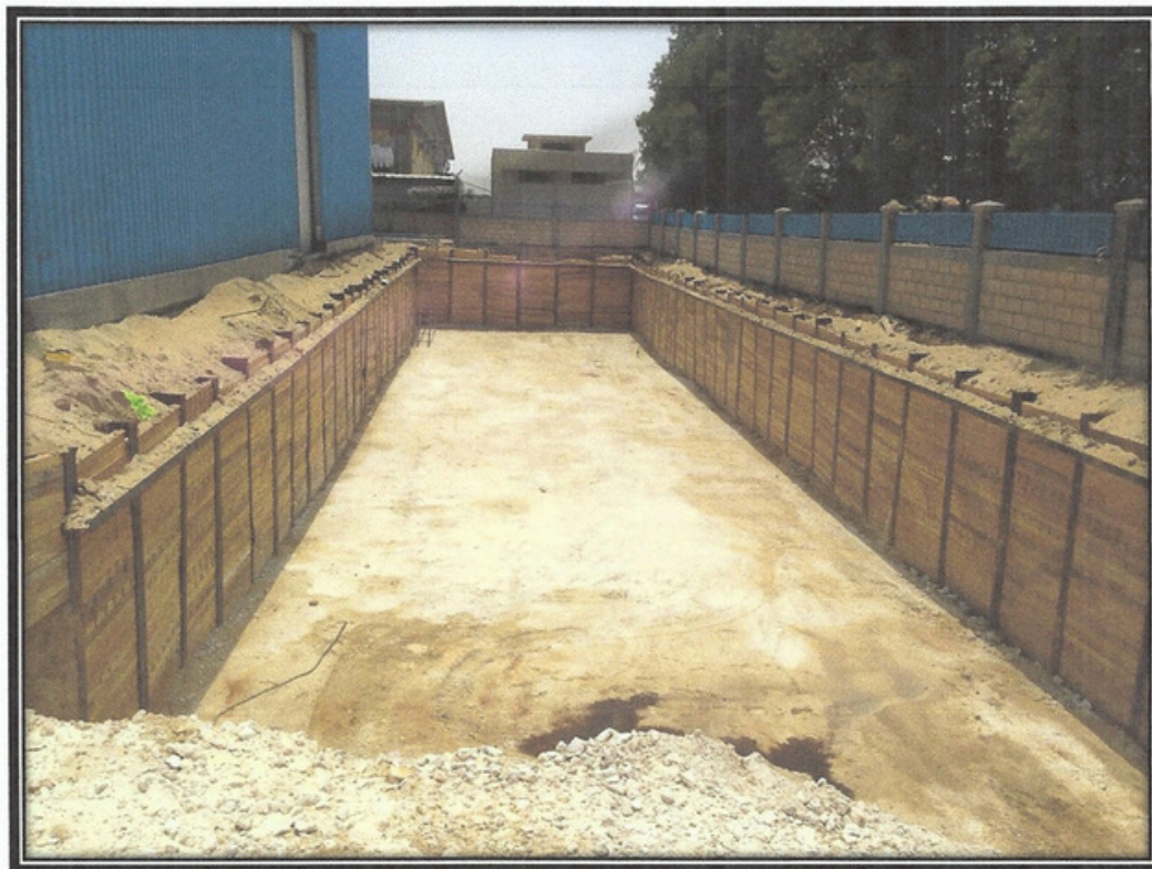
SHORING WORKS AT BASF 2 ND INDUSTRIAL CITY, DAMMAM
