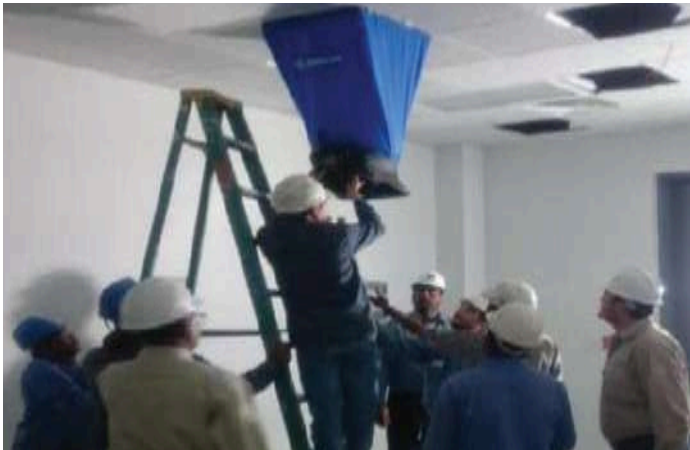
Testing and Air Balancing
