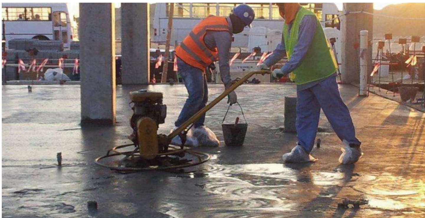
Data Centre Building, Sadara Jubail
