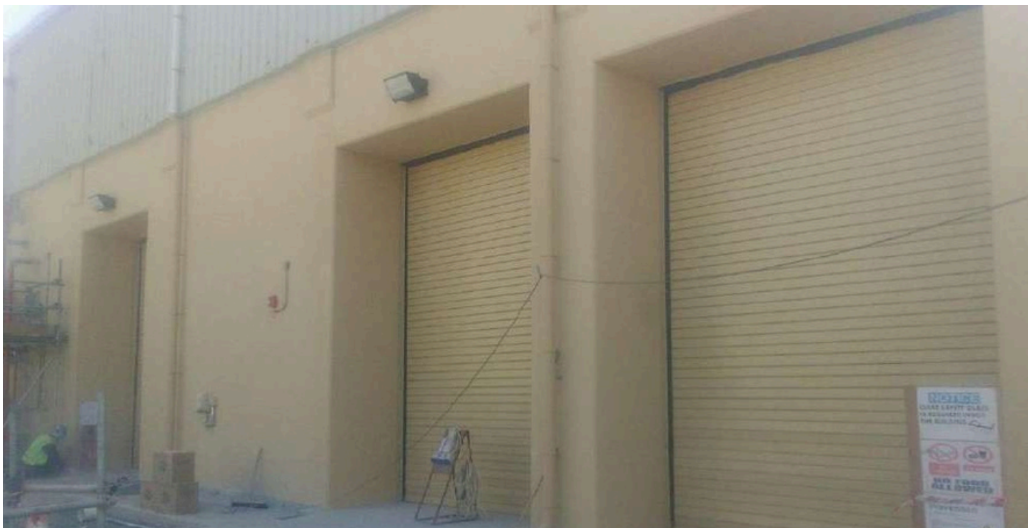
Warehouse & Workshop Building, Jazan IGCC
