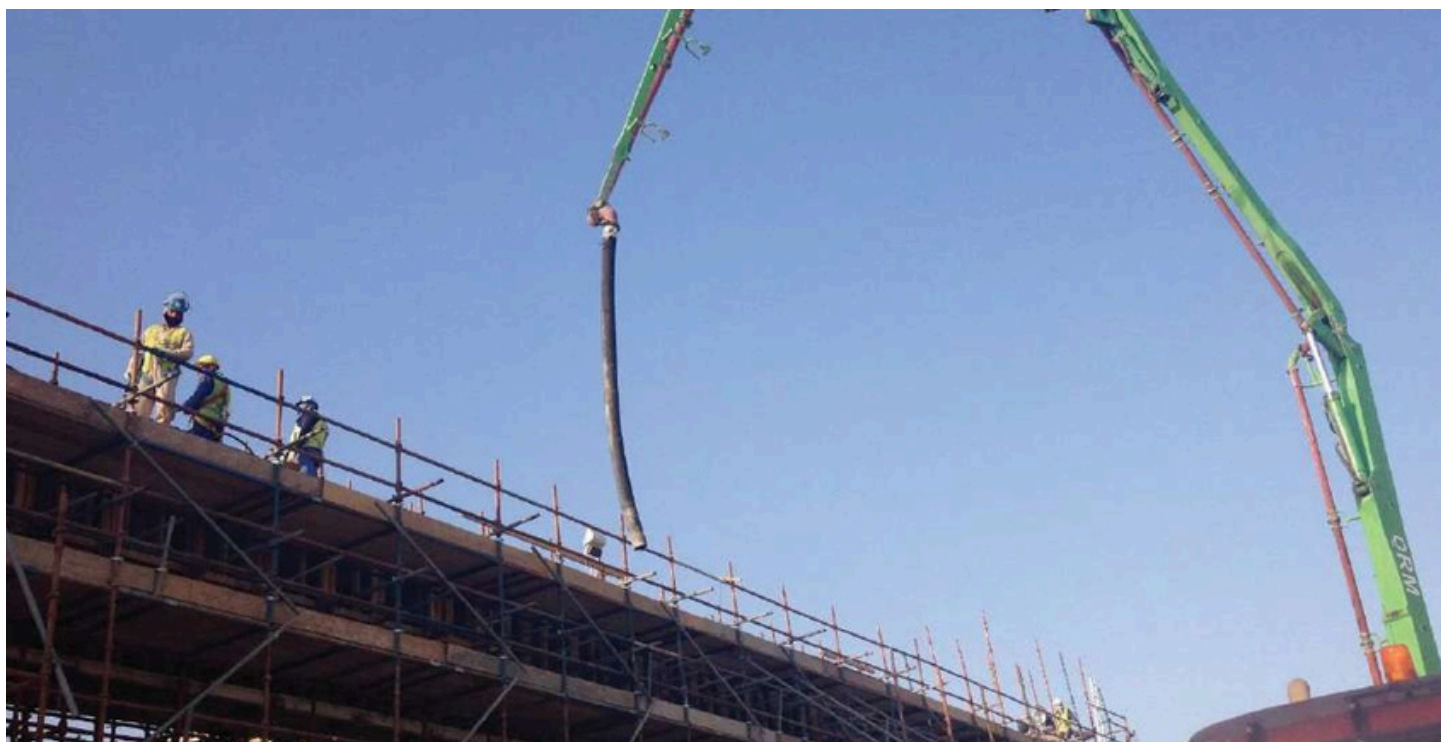
Data Centre Building, Sadara Jubail
