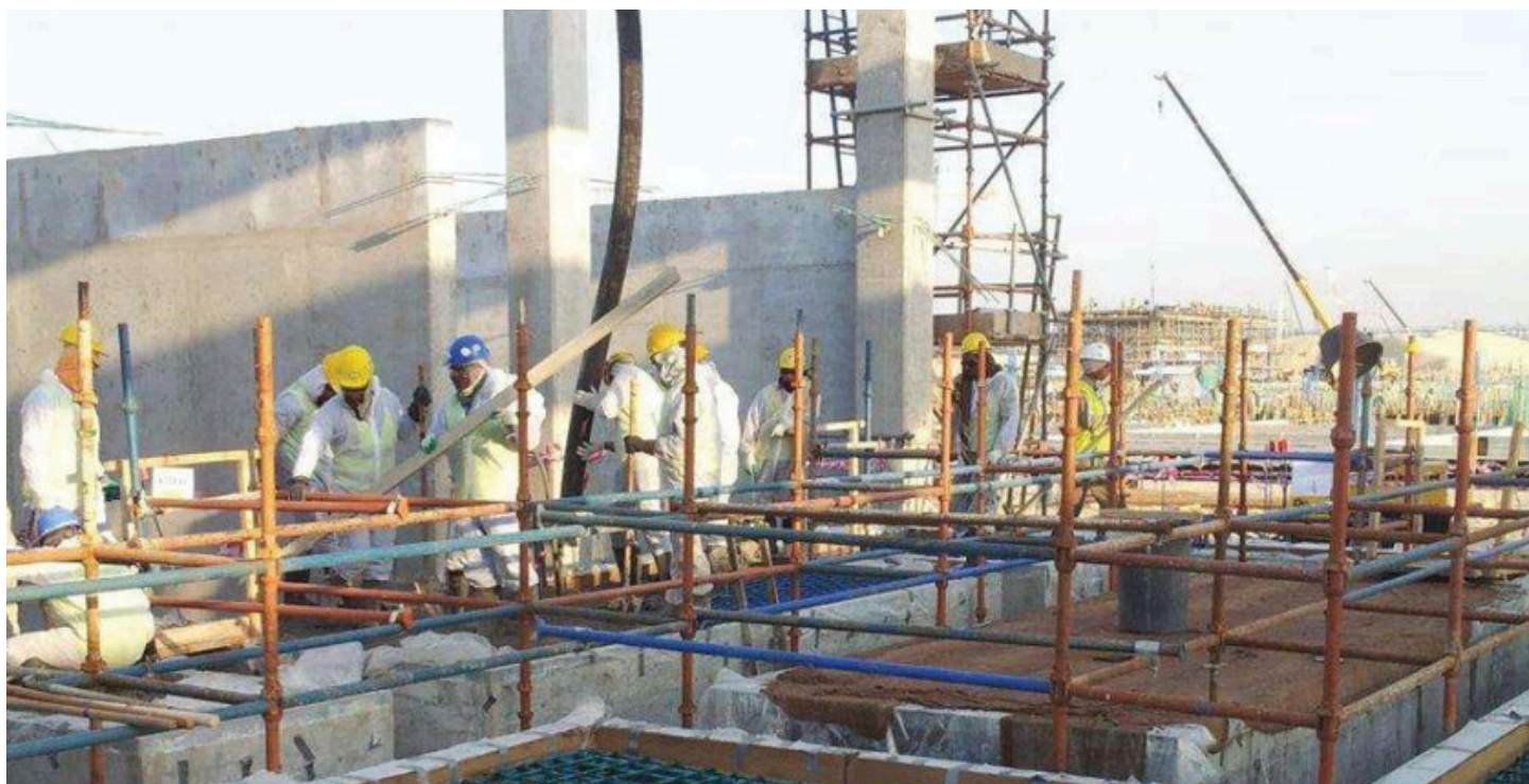
Data Centre Building, Sadara Jubail
