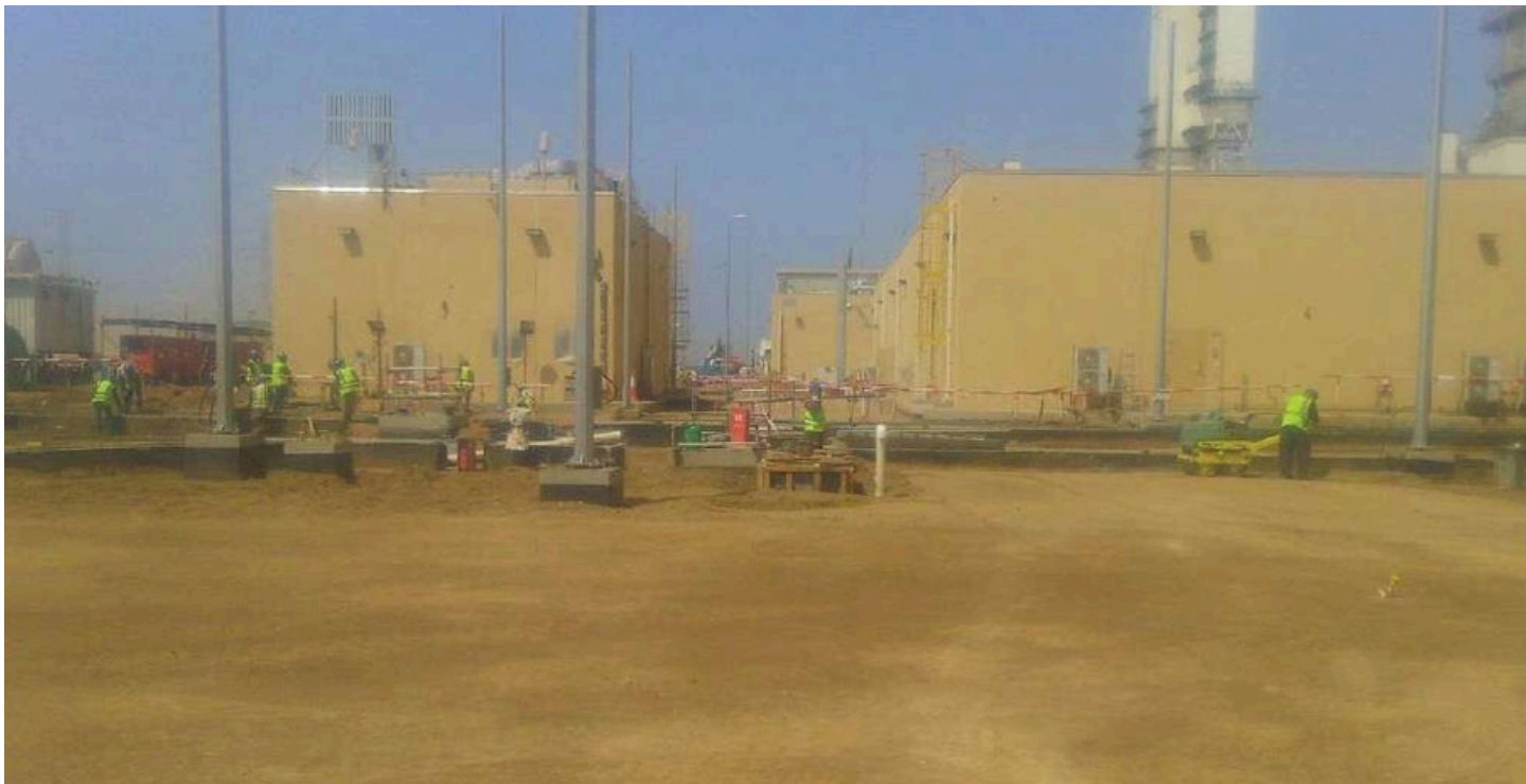
Security & Guard House Building
