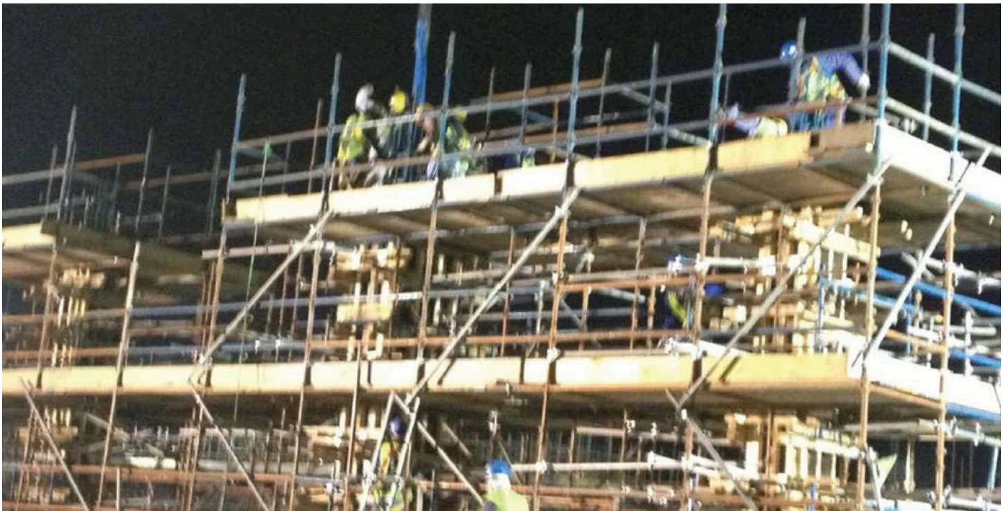
Data Centre Building, Sadara Jubail
