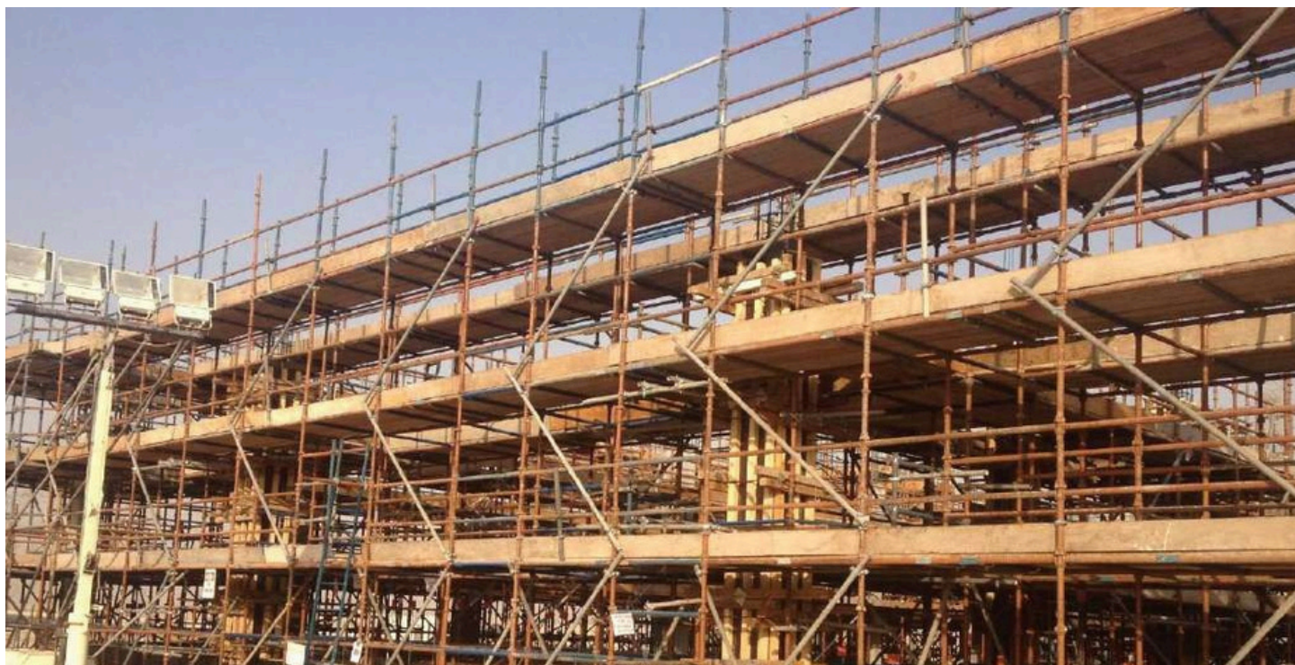
Data Centre Building, Sadara Jubail
