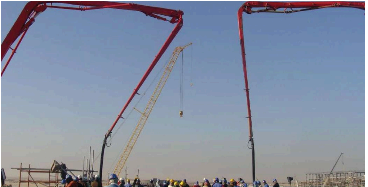
Data Centre Building, Sadara Jubail
