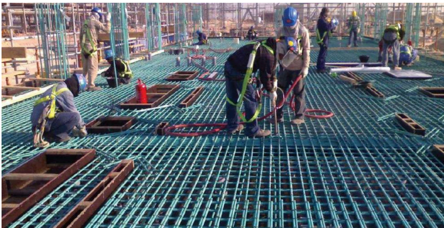
Data Centre Building, Sadara Jubail
