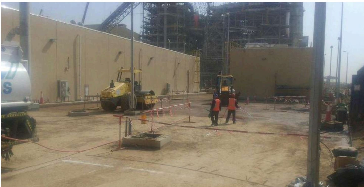
Control Building Site Preparation, Jazan IGCC
