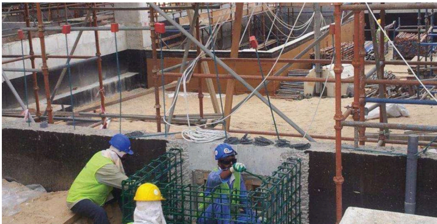
Data Centre Building, Sadara Jubail
