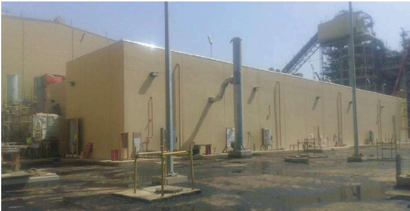
Control & Admin. Building, Jazan IGCC
