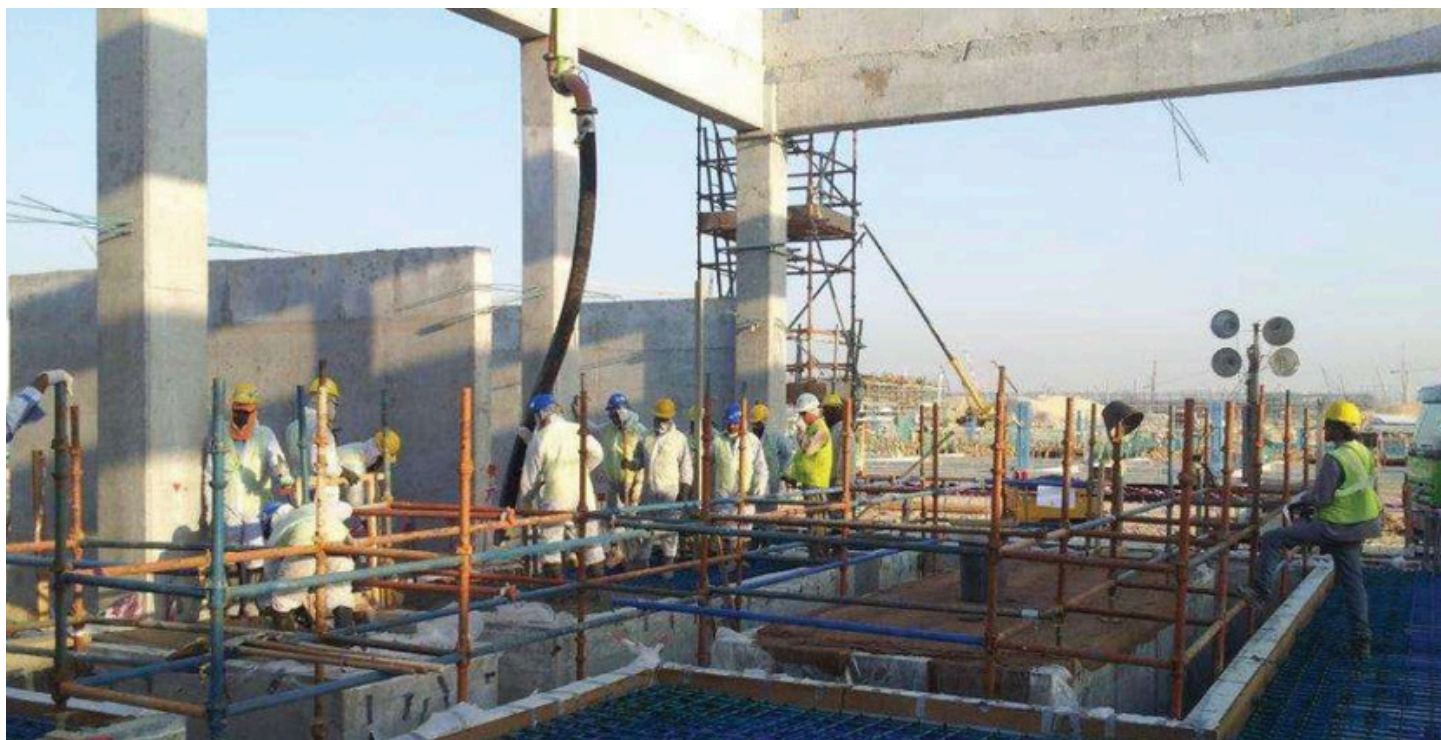
Data Centre Building, Sadara Jubail
