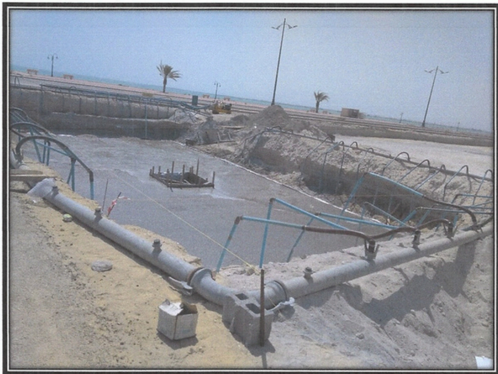
DEWATERING WORKS AT SHUBAILY @ QATIF
