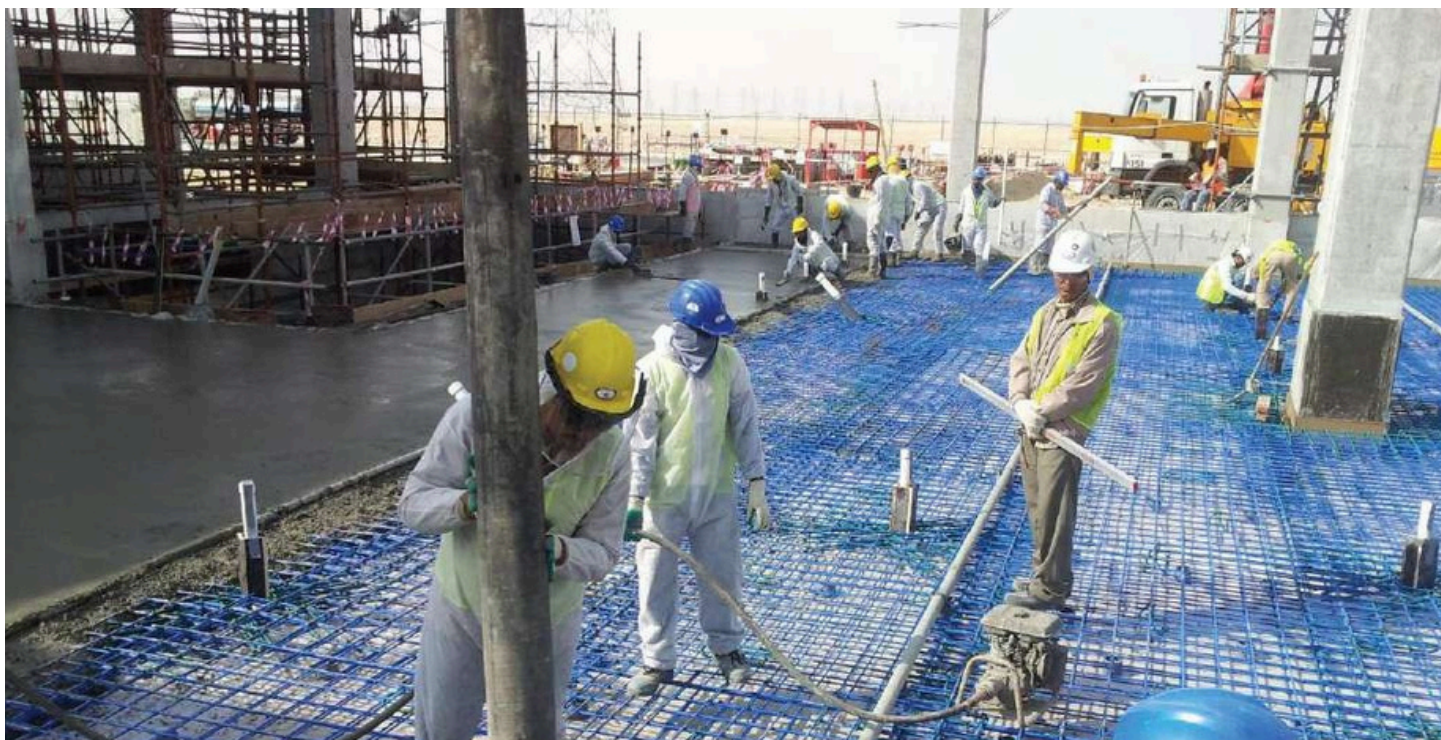
Data Centre Building, Sadara Jubail
